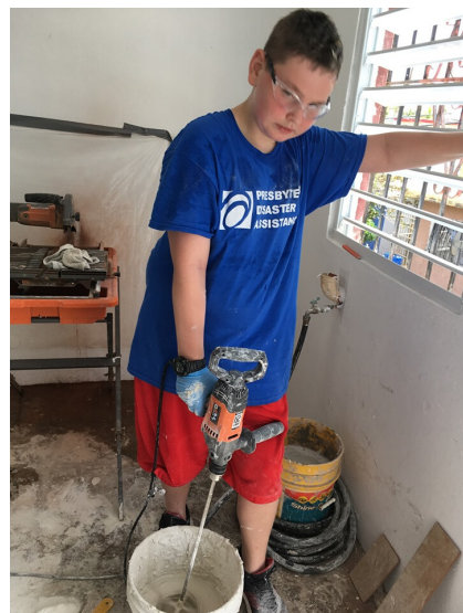
Above: Malachi Calligan mixing and carrying mortar.
